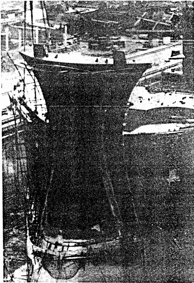
Fig. 71 Tanker bow construction
