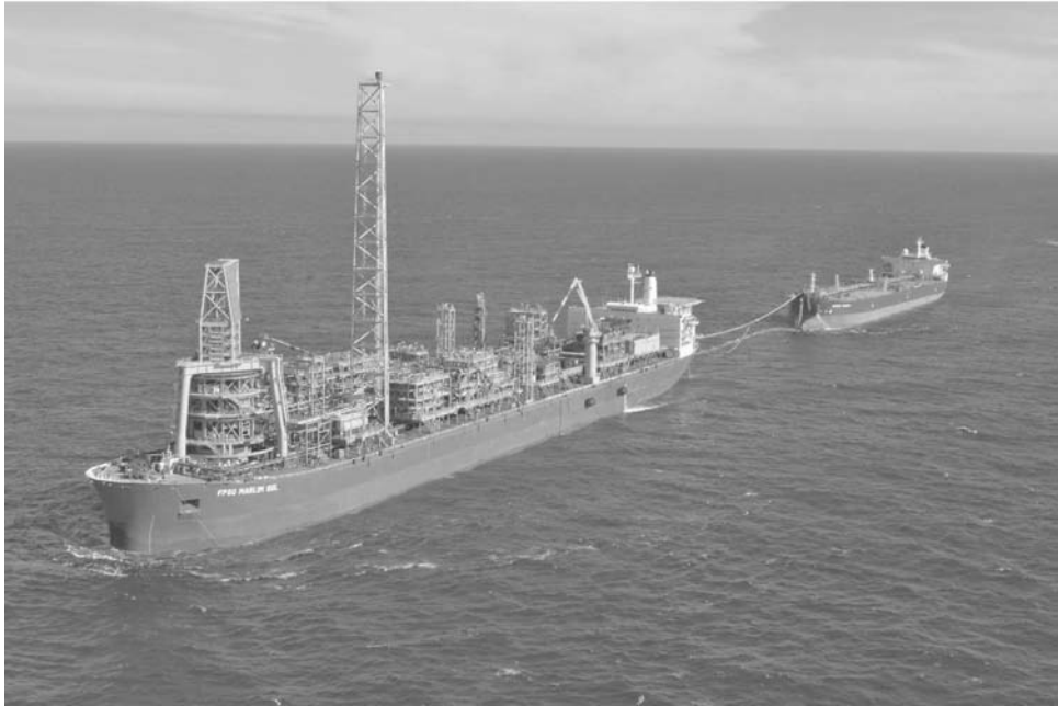
Figure 1.5. (cont.) (d) A photograph of a modern FPSO with an internal turret mooring in a tandem export arrangement (courtesy of SBM Offshore NV).
