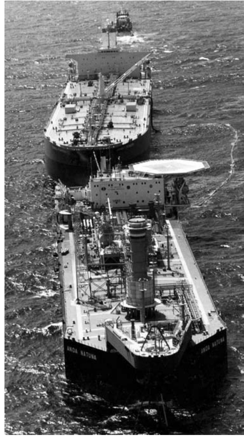
Figure 8.2. Tandem offloading operation of an FPSO (Adhia et al. 2004; courtesy of Society of Petroleum Engineers/Offshore Technology Conference).
