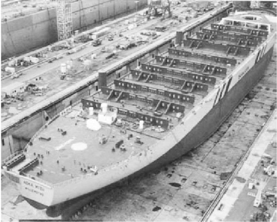
Figure 9.4. A photograph of topside foundation supports consisting of transverse girders, in a ship-shaped offshore unit (Krekel and Kaminski 2002; courtesy of Society of Petroleum Engineers/Offshore Technology Conference).
