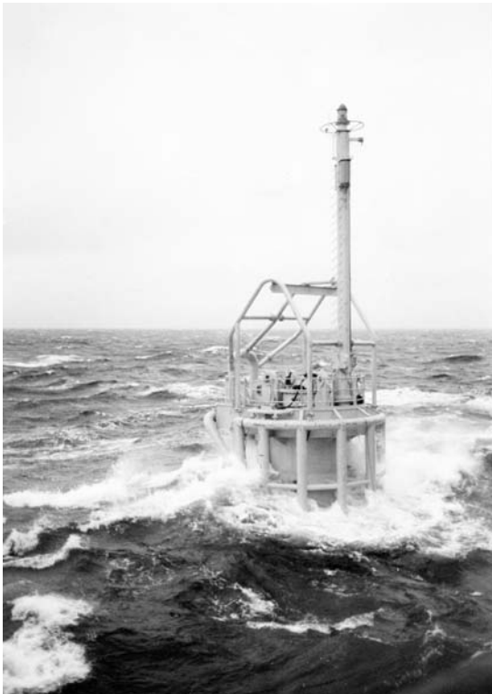
Figure 9.12. (a) An artist's impression of a SALM arrangement with an FPSO (courtesy of SBM Offshore NV). (b) A photograph of a SALM installation (courtesy of SBM Offshore NV).
