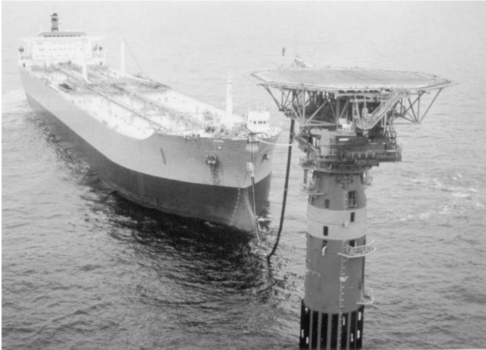
Figure 9.13. A vessel moored at an ALP ready for loading (courtesy of SBM Offshore NV).
