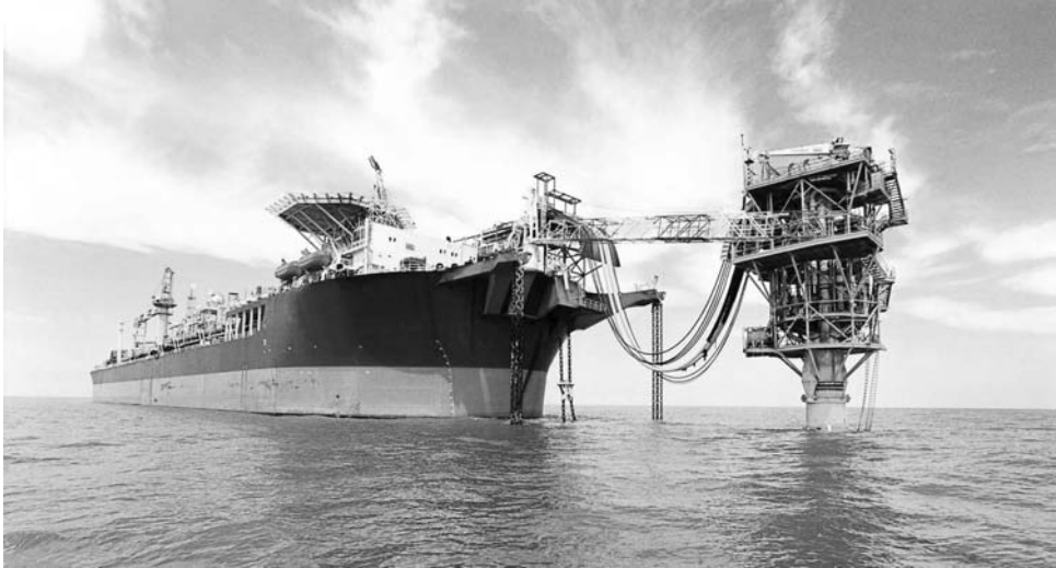
Figure 9.10. A photograph of an FPSO moored at a fixed-tower mooring system (courtesy of SBM Offshore NV).
