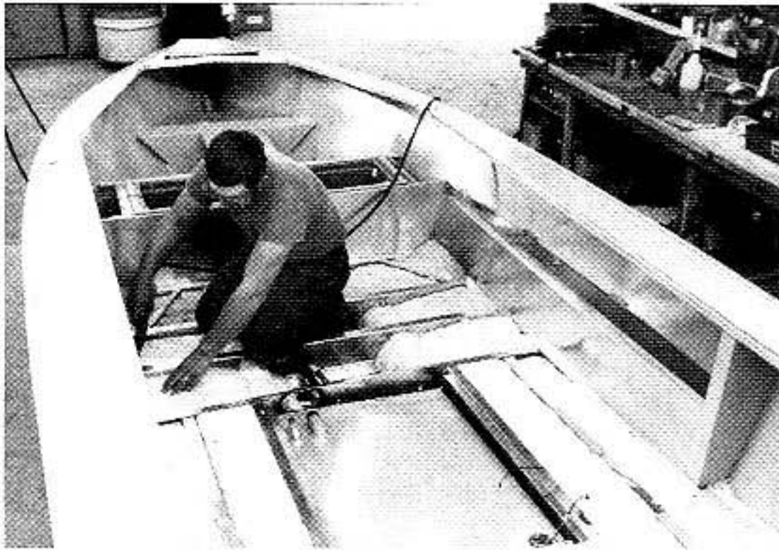
Riveted aluminum-boat assembly. Note the deep floors to support the cockpit sole. Foam flotation and "belly" fuel tank are installed. (Courtesy Lund Boat Company)
