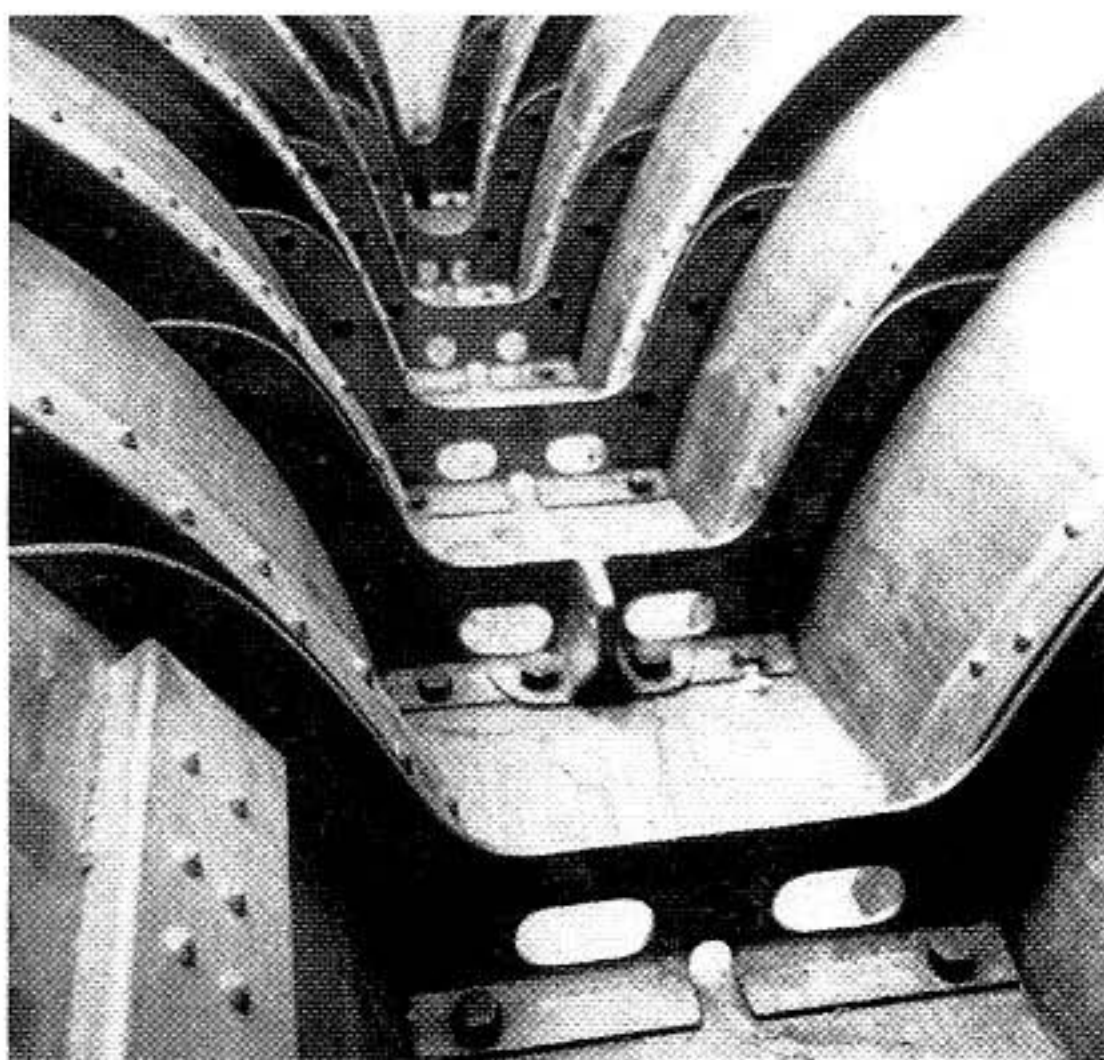
Metal floors installed by Larry and Lin Pardey on their Taleisin. (From Details of Classic Boat Construction: The Hull , by Larry Pardey, reproduced with permission.)
