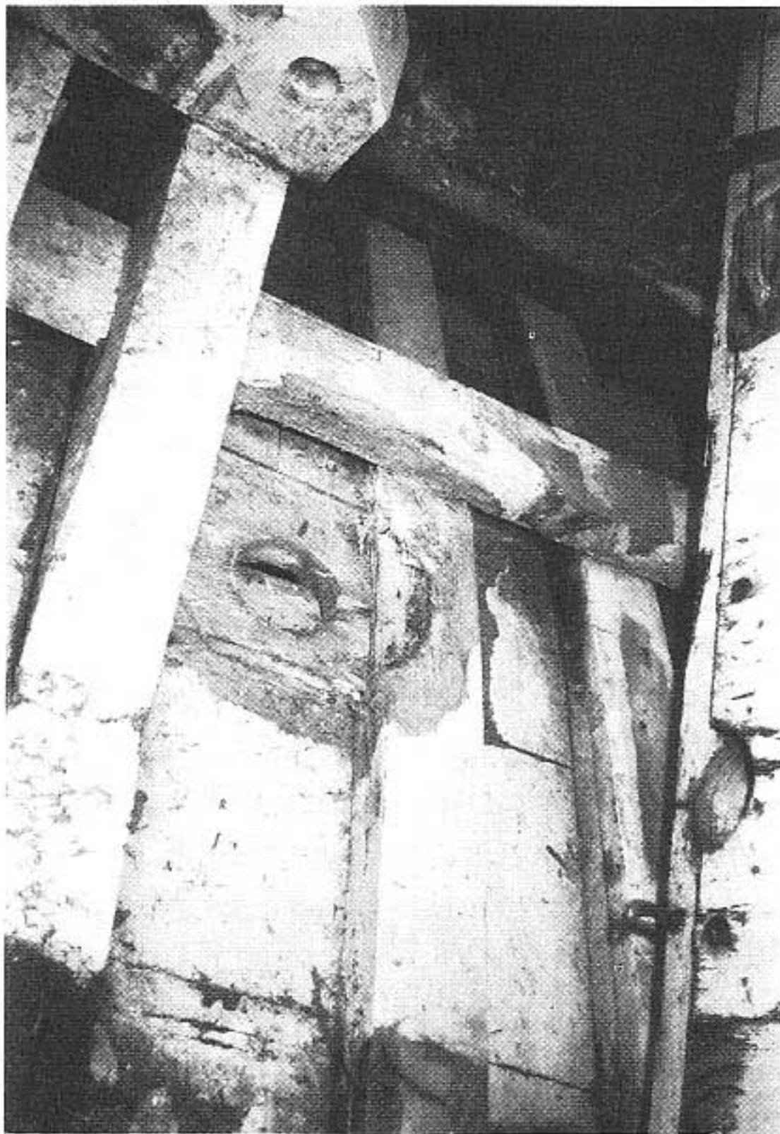
Decay caused by stray current at a through-hull fitting.
