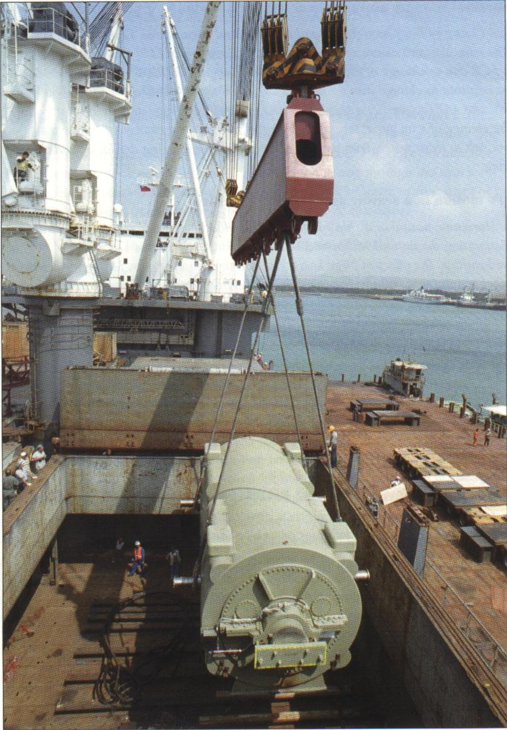
MV Rickmers Tianjin at berth No. 2 Taichuns discharging a 267 T generator unit with ship's gear for a power station project. Special care is needed when handling heavy lifts. See chapter 5.
